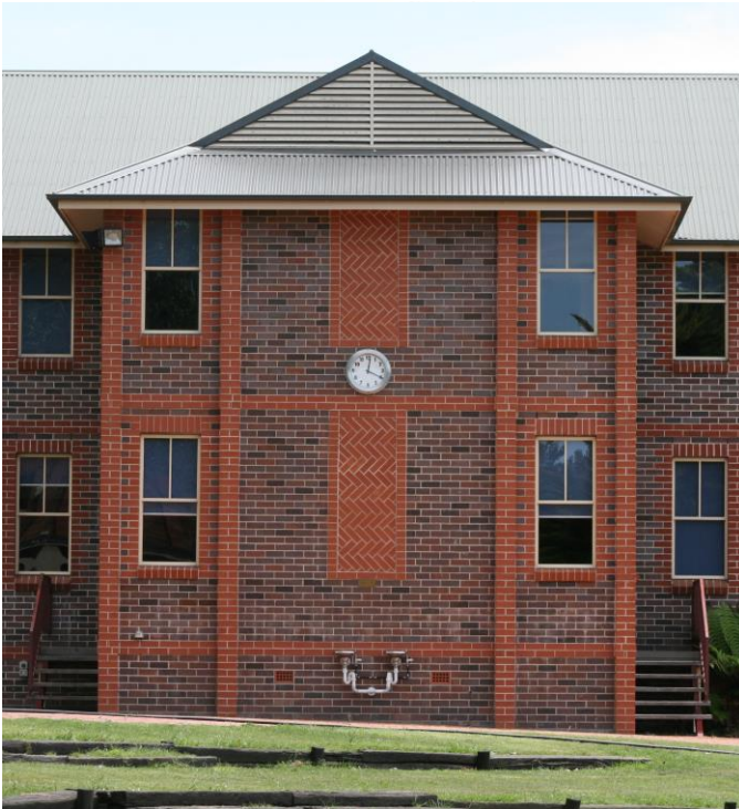
TAS school - Armidale
